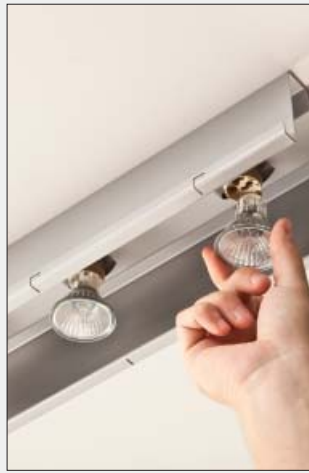
Light bulbs installation
