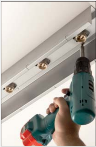
Electrical connection and bar fastening
