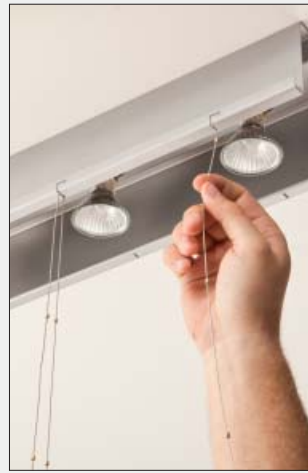
Stainless steel cables insertion and cut
