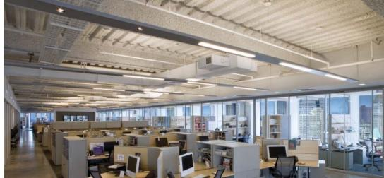
was able to help TPG overcome those challenges by developing customized products to meet specific project needs. One custom fixture, which mounts directly on the ceiling surface, utilizes cleanly detailed extruded aluminum housing and staggered T5 fluorescent lamps to create an unbroken line of light. Another is a pendant luminaire that features both T5 and MR16 components in steel housing with a slender profile.
